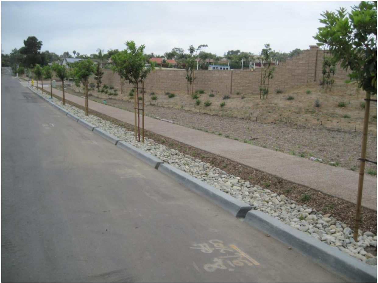
Figure A.4-1. Rock Infiltration Swale.
